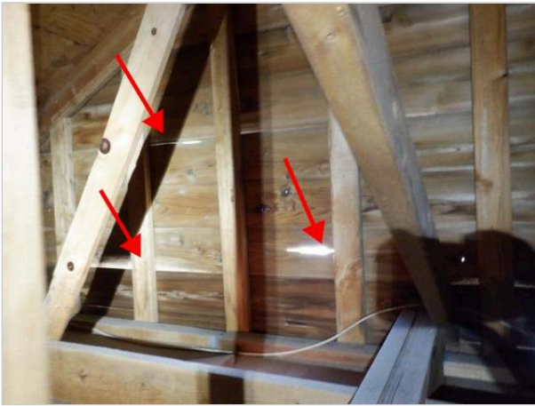
Daylight at front gable
