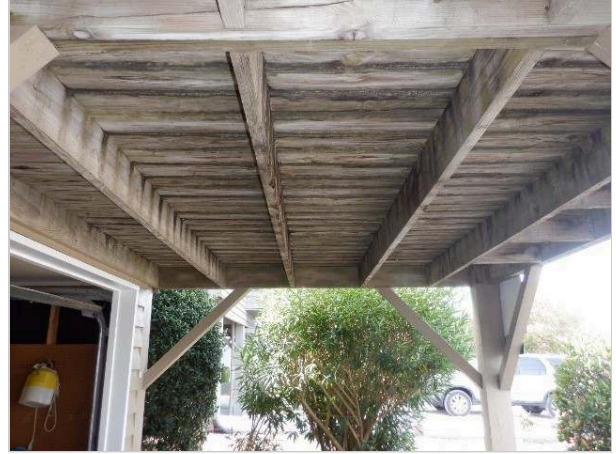
Joists 24" on center
