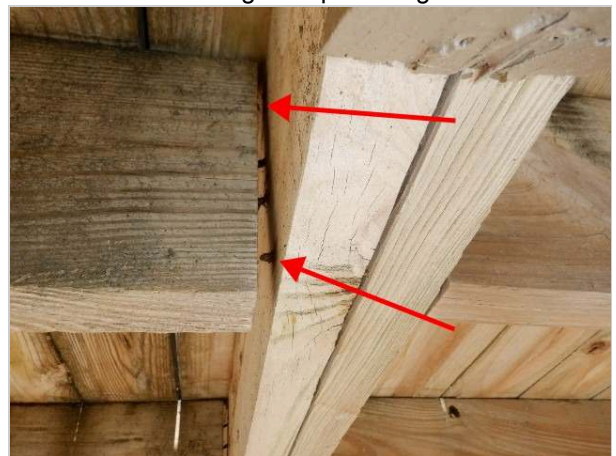
Corroded nails
