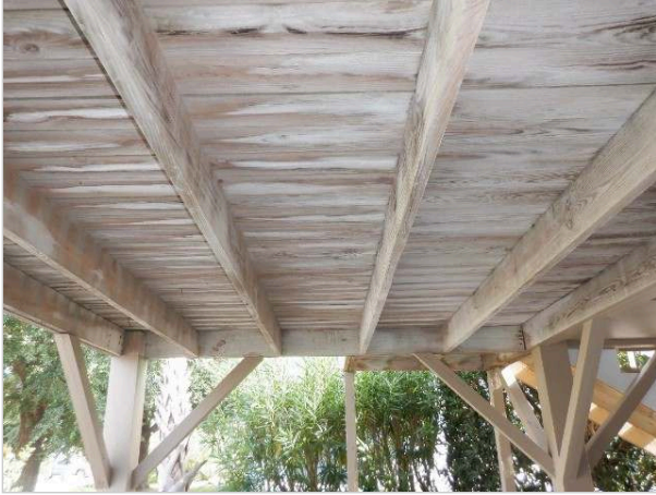
Joists 24" on center
