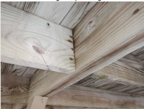
Corroded nails
